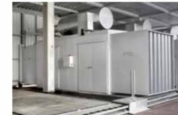
**'Dry' exhaust gas systems** Despite the space problems in the generator set, Discom is perfectly capable of designing 'dry' exhaust systems that will meet your requirements. We design and manufacture 'dry' silencers in different shapes. In doing so we guarantee optimal use of volume and good acoustic results while respecting the maximum permissible back pressure in the exhaust system. In most cases we provide an integrated and certified spark arrestor.
